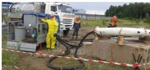
Flushing the pipeline hot solutions
